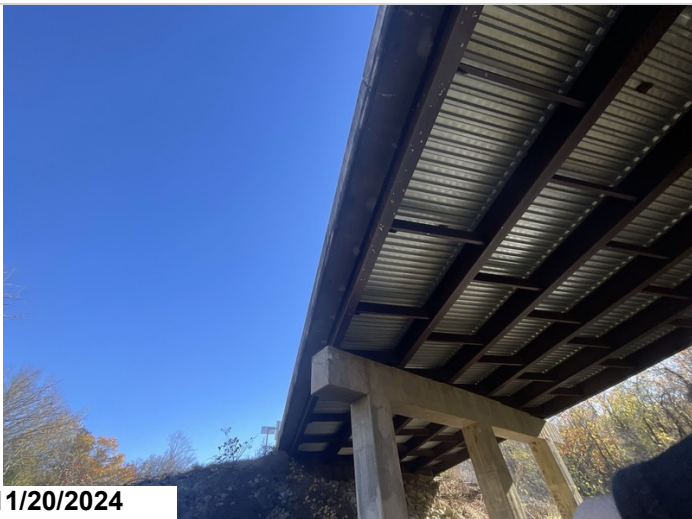
Typical overhangs have 8SF CS2 PER side per span. 48SF CS2
