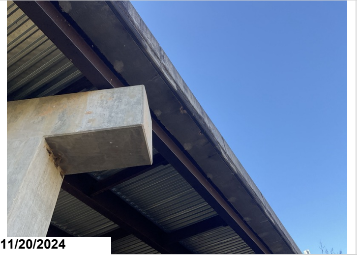
Span 3, right: has 2 spalls with exposed rebar. 2' CS3
