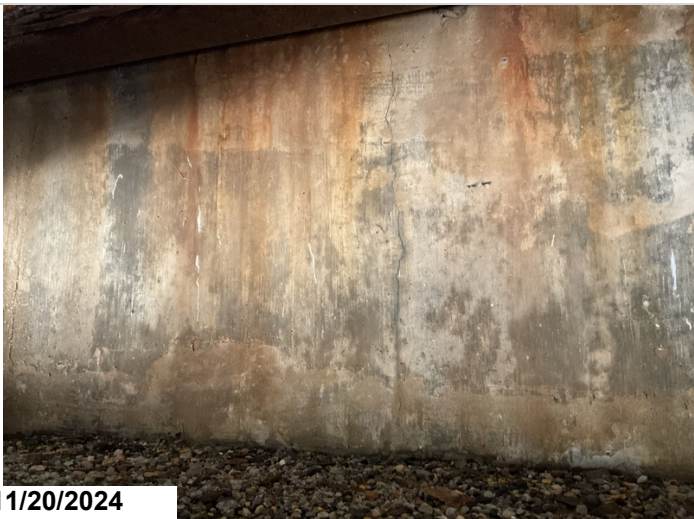
Typical cracks to backwall.
