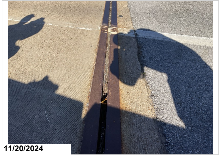
Abutment 1, seal. Both all in CS3. 94' CS3
